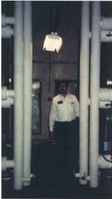
An exterior view of the chilled water coil chamber.
