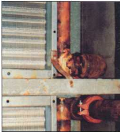
A perfect fit! The close tolerance for the supply and return lines was no problem for Heatcraft manufacturing and assured the job would be completed on time - saving the hospital big dollars.
