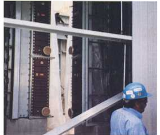
Typical installation of the completed coil and drain pans as designed and fabricated by Heatcraft.
