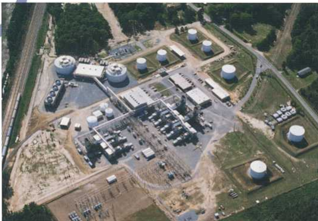
Photo courtesy of Burns & McDonnell
